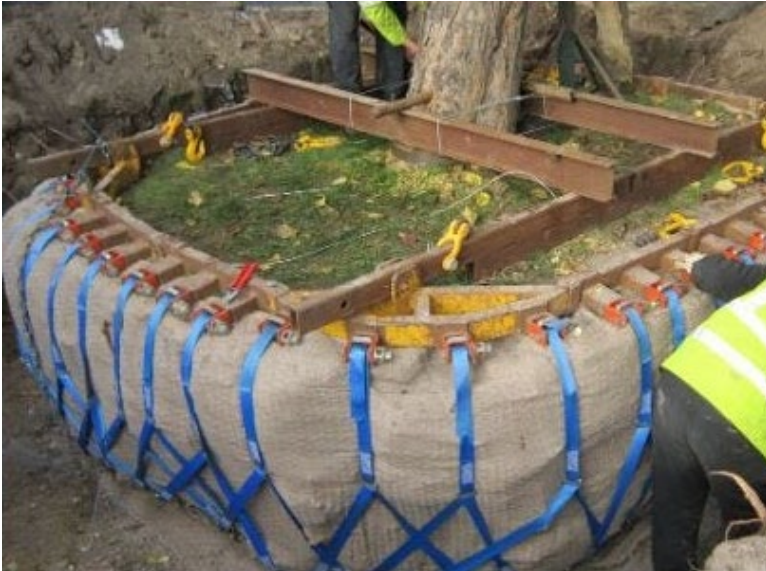
Image of prepared root ball prior to lifting.
